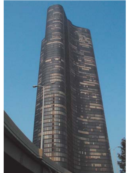
A McQuay dual compressor centrifugal chiller provides quiet operation and energy cost savings for Harbor Point Condominiums in Chicago.
